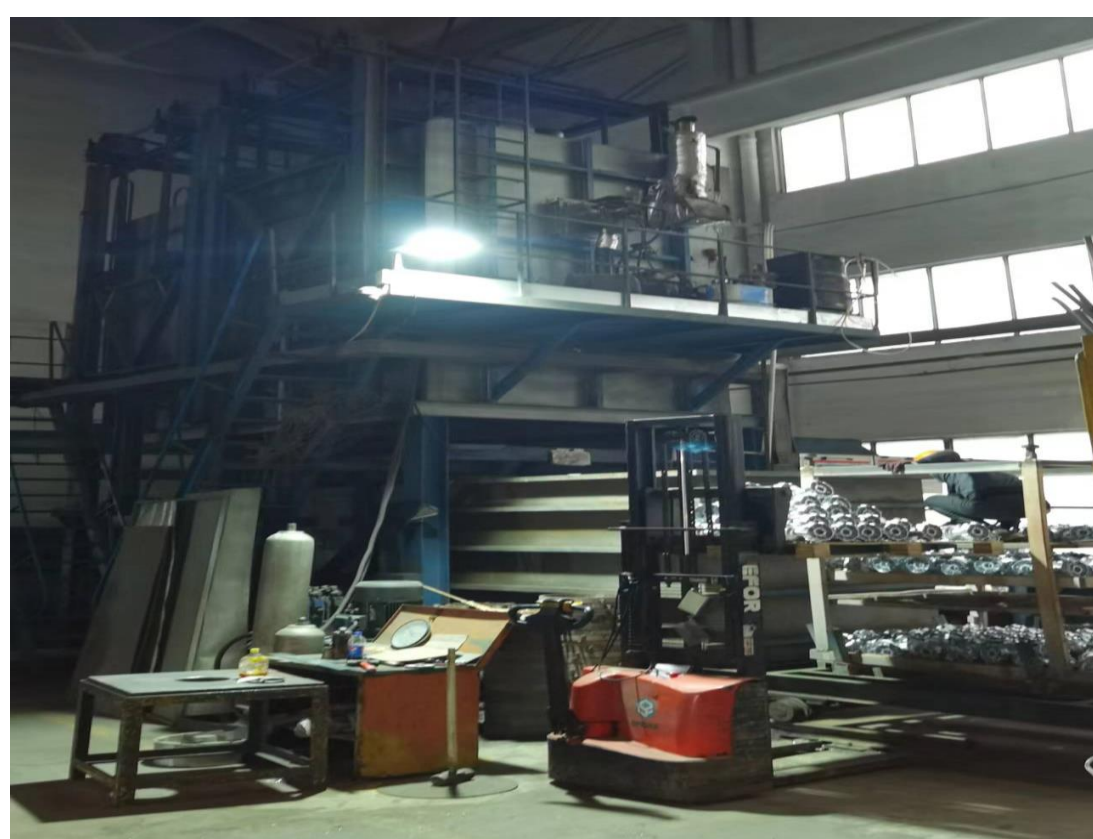
固溶炉 Solid solution furnace
